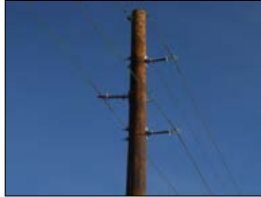
Figure 5-18. Vertical tangent unit (grounded).
