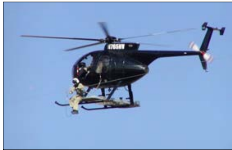
Figure 8-6. Marker installation by helicopter.
