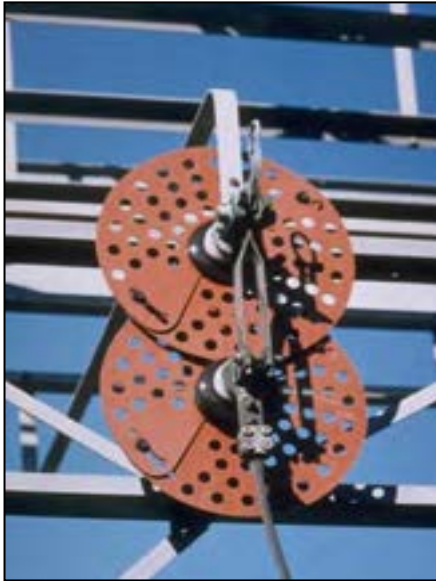
Figure 5-78. Barrier plate on switch (TE Connectivity).
