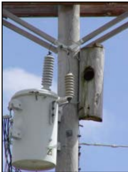
Figure 9-22. Active woodpecker nest accommodated during pole replacement.
