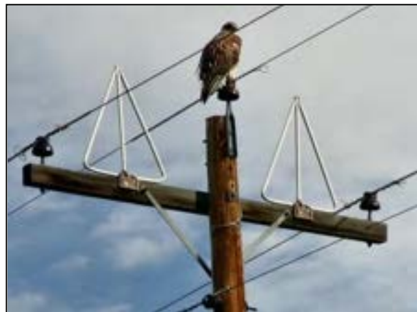
Figure 5-104. Perch discourager shifting a raptor to the pole top.
