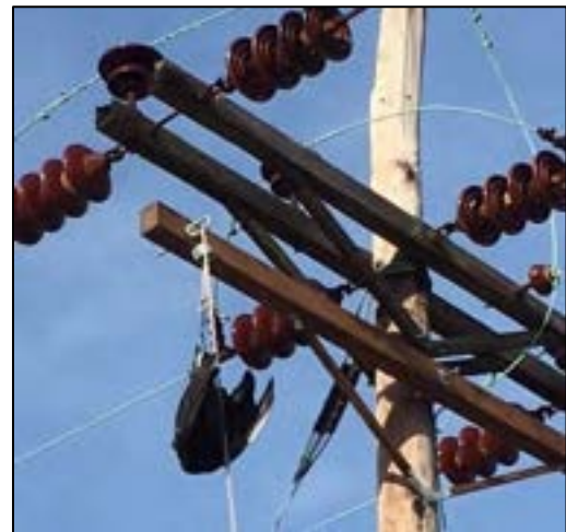
Figure 5-117. An effigy can reduce or eliminate substation roosting by Black Vultures and Turkey Vultures (Cristina Frank).
