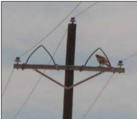
Figure 5-106. Raptor perching beneath a perch discourager.
