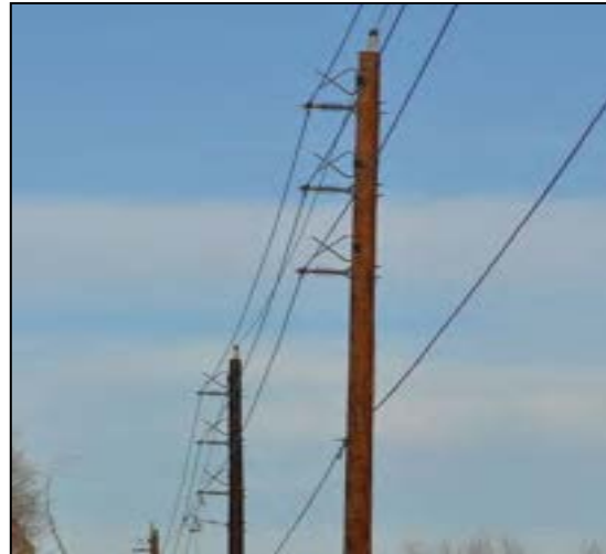
Figure 5-24. Isolating each phase with a perch discourager (Power Line Sentry).
