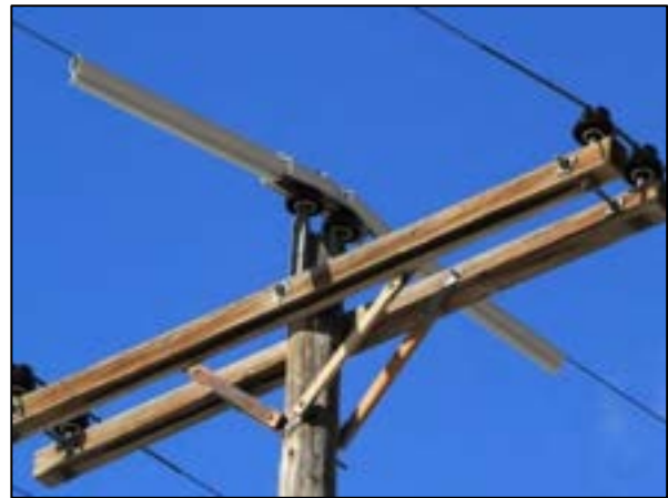
Figure 5-15. Power Line Sentry, LLC conductor cover.
