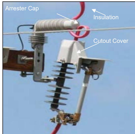
Figure 5-50. Protected cutout/arrester combination.
