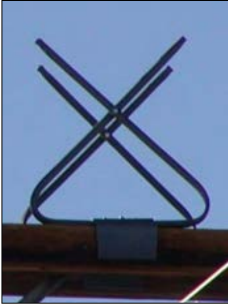
Figure 5-101. Power Line Sentry "Raptor Guard" perch discourager design to deter perching within the triangle.
