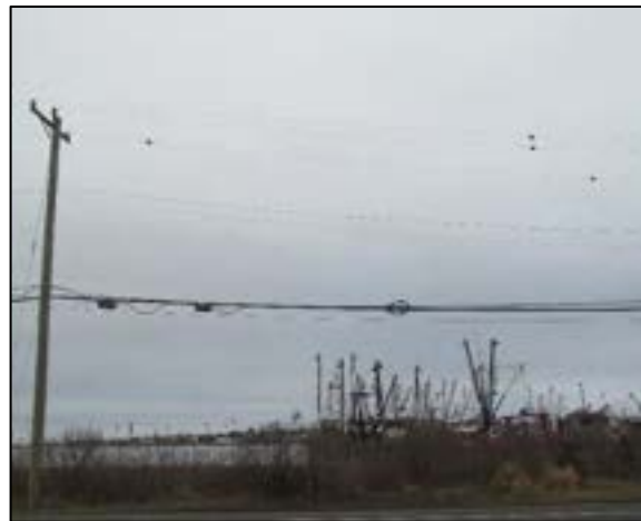
Figure 8-27. Previous generation passive markers could migrate toward the lowest point in the span.
