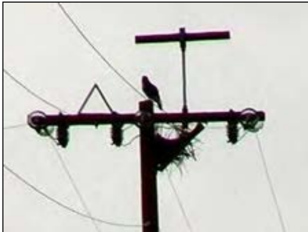
Figure 5-98. Raptor perching below an elevated perch.
