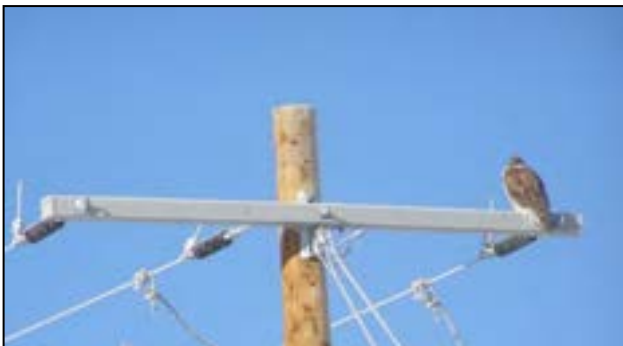
Figure 9-24. Fiberglass deadend single crossarm.
