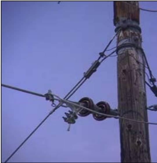
Figure 5-91. Guy wires attached to grounded pole bands.
