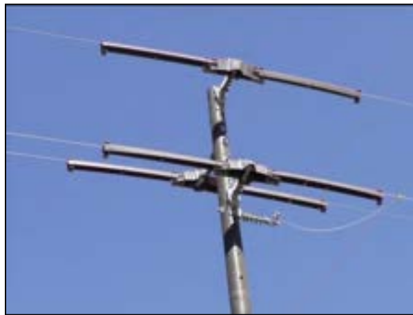
Figure 5-22. Three conductor covers are required for adequate protection on a steel pole (TE Connectivity).
