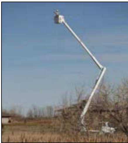
Figure 8-5. Marker installation by bucket truck.
