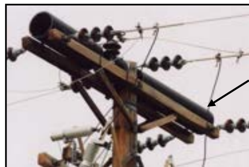
Figure 9-19. Homemade conduit stick deflector.
