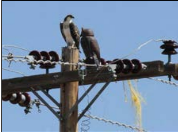
Figure 5-115. Plastic owl unsuccessfully preventing perching.
