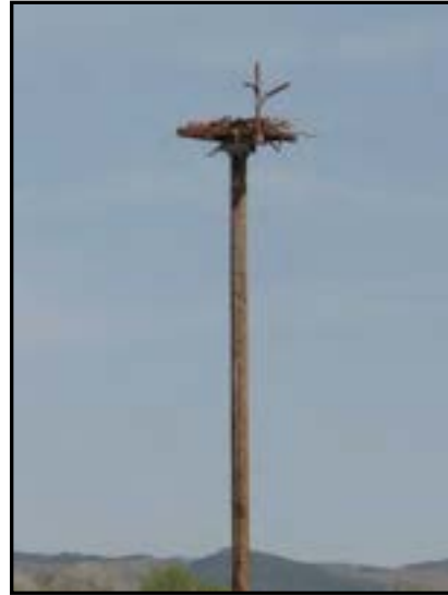
Figure 9-5. Nesting platform on a surrogate pole.
