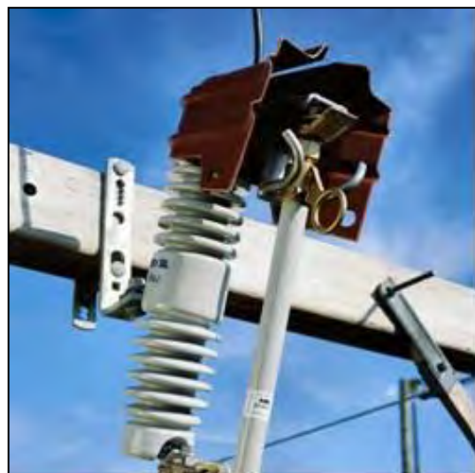
Figure 5-51. Cutout cover (TE Connectivity).
