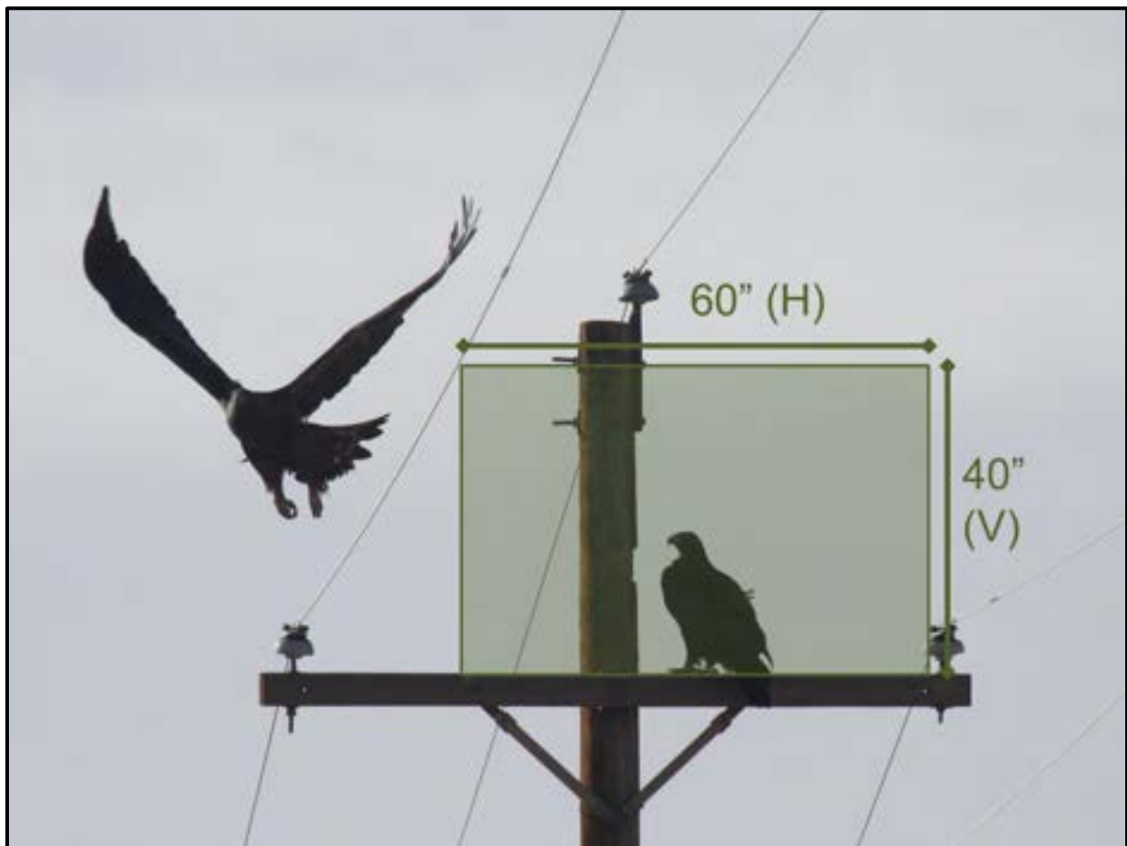
Figure 5-1. Recommended APLIC clearances to minimize electrocution risks.
