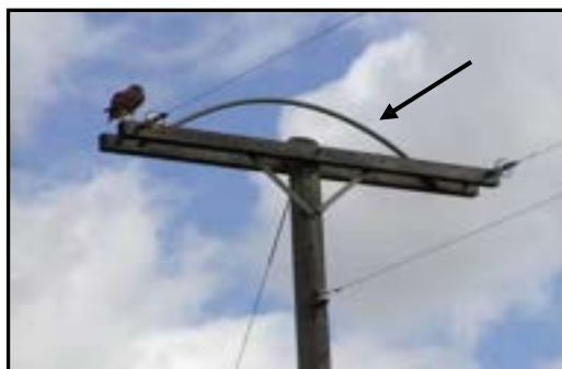
Figure 9-18. Homemade PVC stick deflector.
