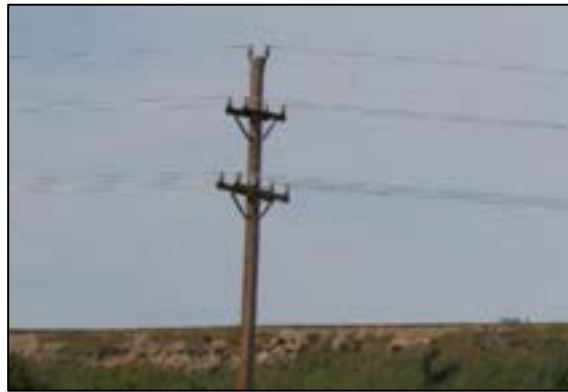
Figure 8-29. Flat T2 conductor appears to move downline as it twists in the wind.
