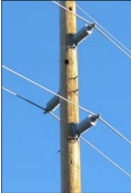
Figure 6-3. Avian-friendly vertical configuration with ungrounded insulator bases.
