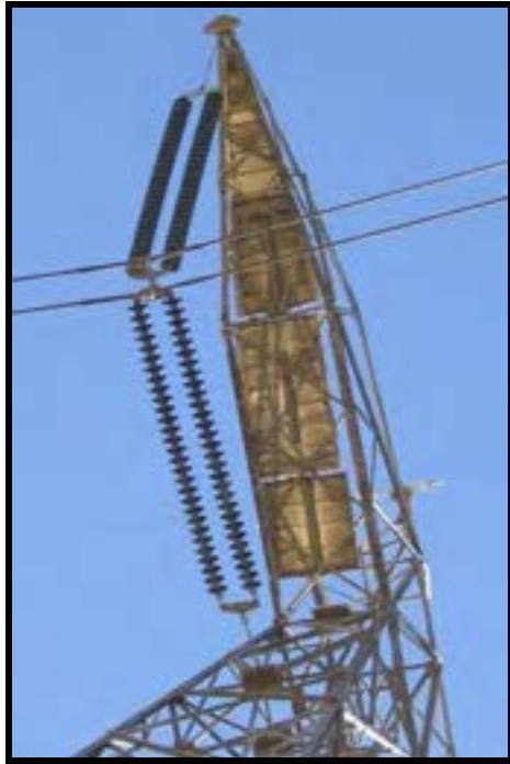
Figure 10-12. Lattice structure with contamination shields (Zena).
