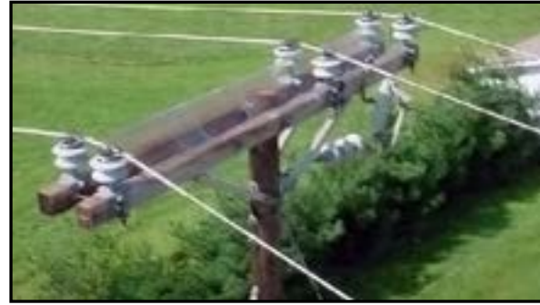
Figure 9-15. Stick deflector (Utility Solutions, Inc.).
