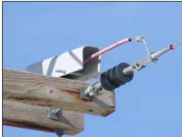
Figure 5-39. Jumper isolated with a pin cover.
