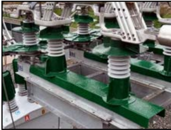
Figure 7-16. Switch with custom-formed barrier plates (Cantega Technologies, Inc.).
