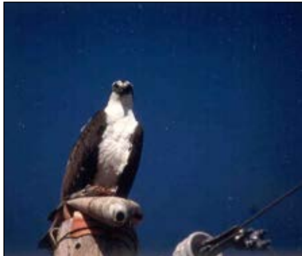
Figure 5-107. Inappropriate use of a traffic cone as a perch discourager (Chad Olsen).
