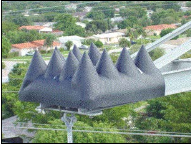
Figure 10-1. HDPE cones deployed on the arms of a lattice transmission structure (Zena Design).
