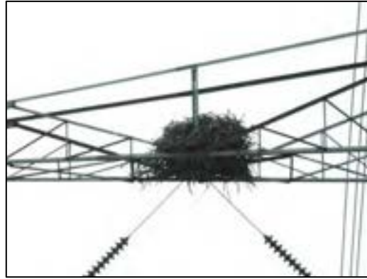
Figure 2-24. Bald Eagle nest on a steel lattice transmission structure.
