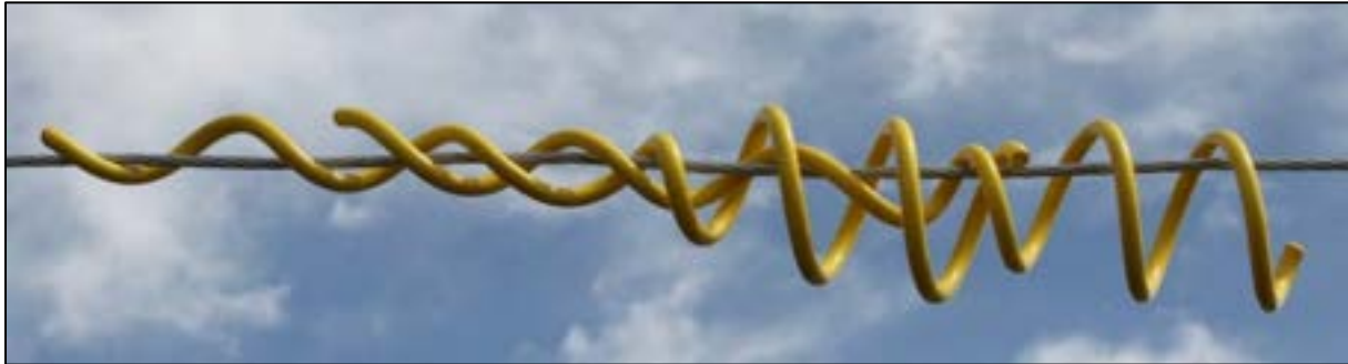
Figure 8-25. Improperly installed markers that have shifted.
