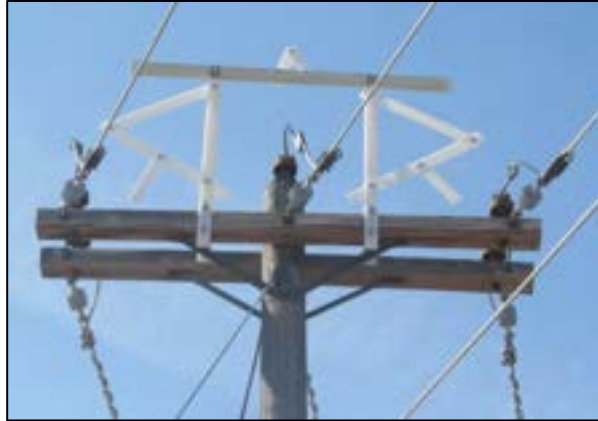
Figure 5-97. Elevated perch (Bird Powerline Protection Ltd.).
