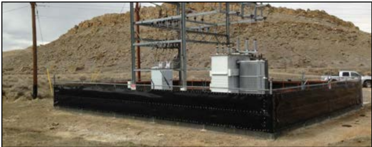
Figure 7-18. Animal-exclusion fence constructed to exclude rodents.
