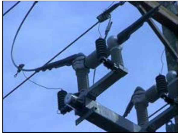
Figure 5-82. Switch with built-in animal protection.
