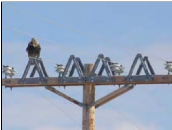
Figure 5-103. Bird perching on a perch discourager.
