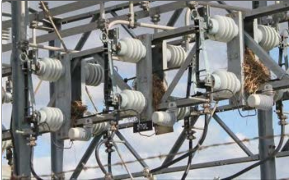
Figure 2-8. Nesting birds may attract larger predators to a substation, increasing the electrocution risk.
