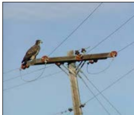
Figure 5-26. Three-phase double deadend with jumpers routed under the crossarms (center phase still needs deadend covers).
