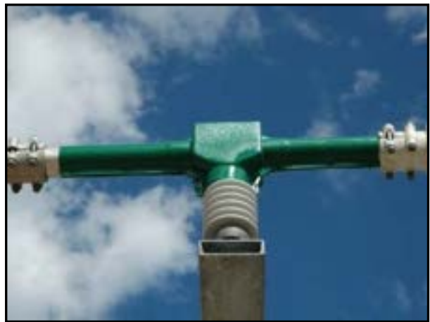
Figure 7-5. Form-fitted bus insulation (Cantega Technologies, Inc.).
