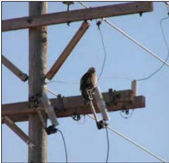
Figure 5-49. Hawk perched between unprotected cutouts and arresters.
