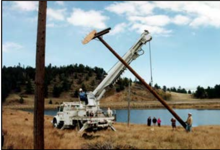
Figure 9-11. Raptor platform with pegs.
