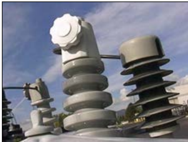
Figure 5-41. “Wheel-type” bushing cover from the manufacturer.
