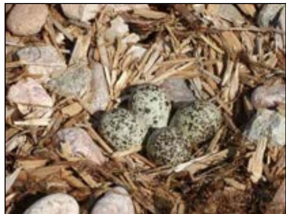
Figure 2-27. Killdeer nest within a substation.
