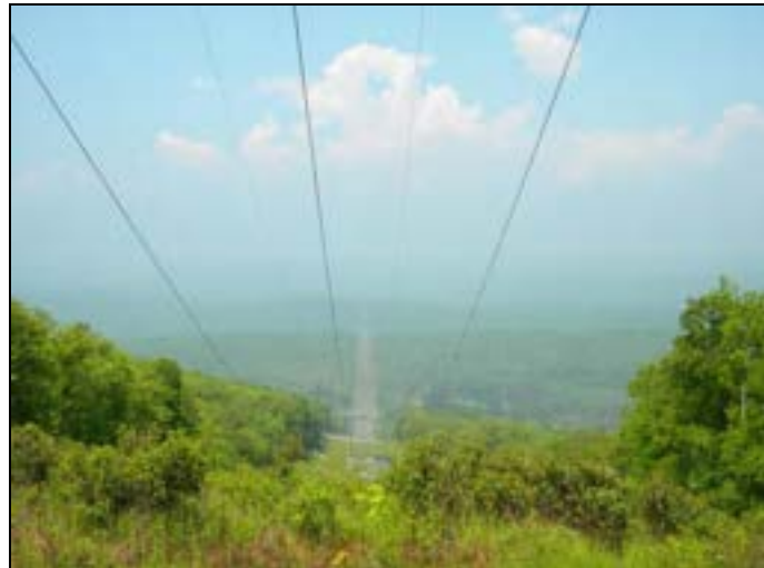
Figure 2-16. OHS wires are less visible than conductors.
