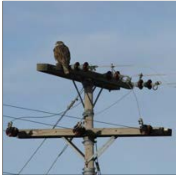
Figure 5-92. Guy wires attached to grounded pole bands.
