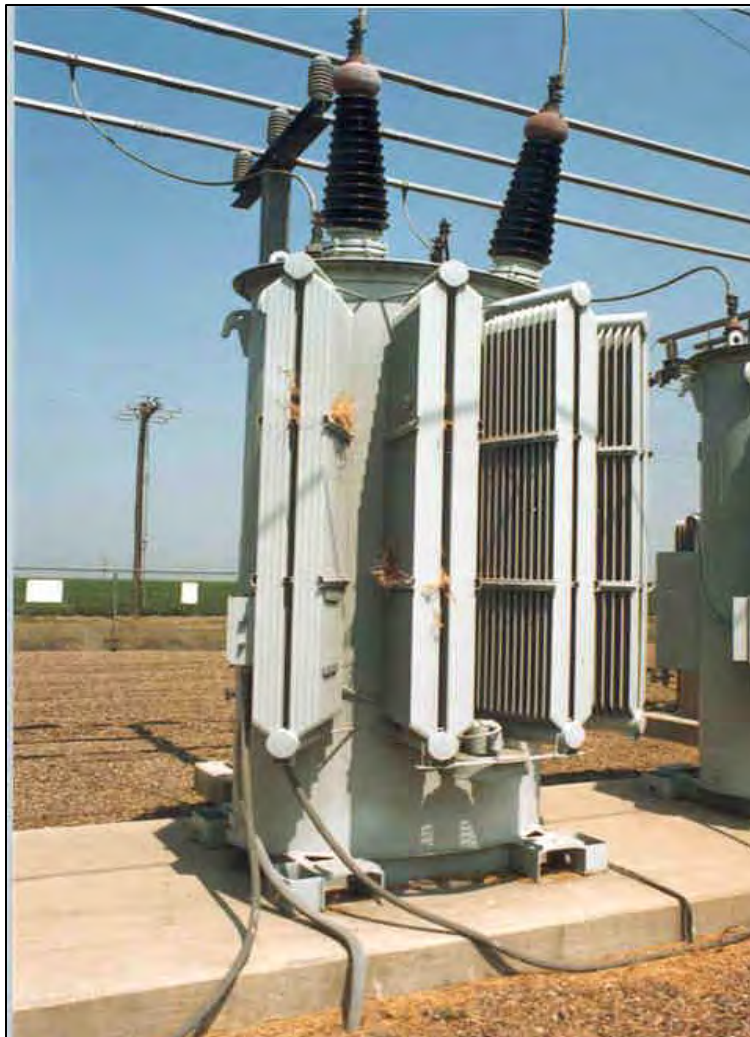
Figure 2-9. Nests in substation transformer cooling fins (EPRI).
