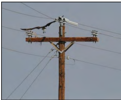
Figure 5-10. A typical ridge-pinned tangent structure retrofitted with conductor covers (Power Line Sentry, LLC).
