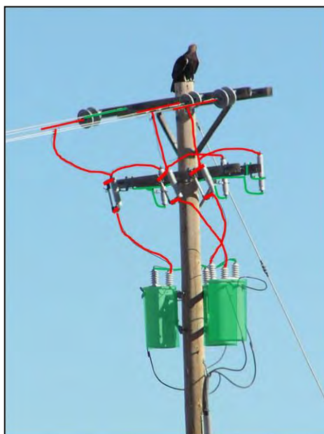
Figure 2-4. Complex transformer pole with many jumper wires, and little separation between energized (red) and grounded (green) contacts.
