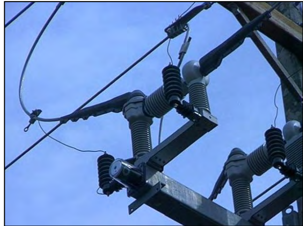
Figure 5-82. Switch with built-in animal protection.
