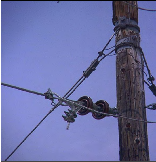
Figure 5-91. Guy wires attached to grounded pole bands.
