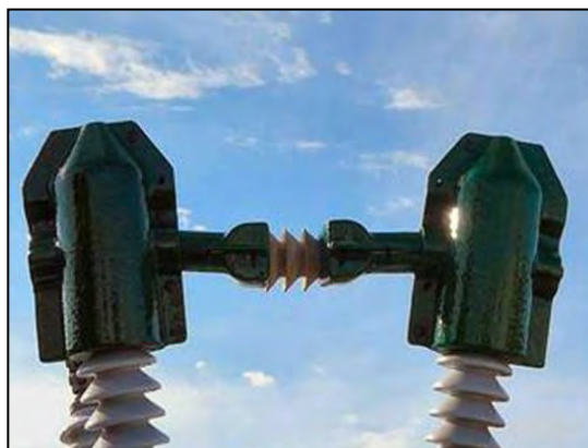
Figure 5-77. Regulator with bypass arrester cover. (Photo credit: Cantega)
