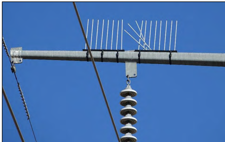
Figure 10-3. Raptor Guard Spike Perching Excluders with angled spikes to block perching above insulators (Power Line Sentry, LLC).
