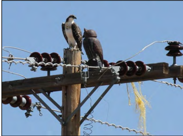
Figure 5-115. Plastic owl unsuccessfully preventing perching.
