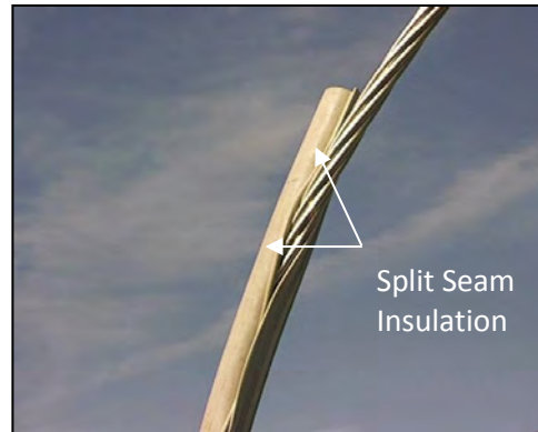
Figure 5-35. Split-seam stinger retrofit (Salisbury insulating SALCOR cover material).
