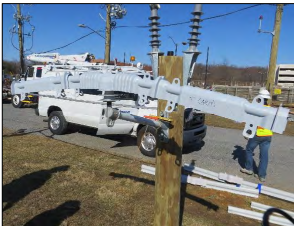
Figure 5-14. Hendrix Molded Products conductor cover.
