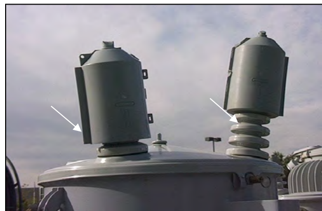
Figure 5-44. Hubbell Power Systems, Inc. bushing covers installed incorrectly (left) and correctly (right).
