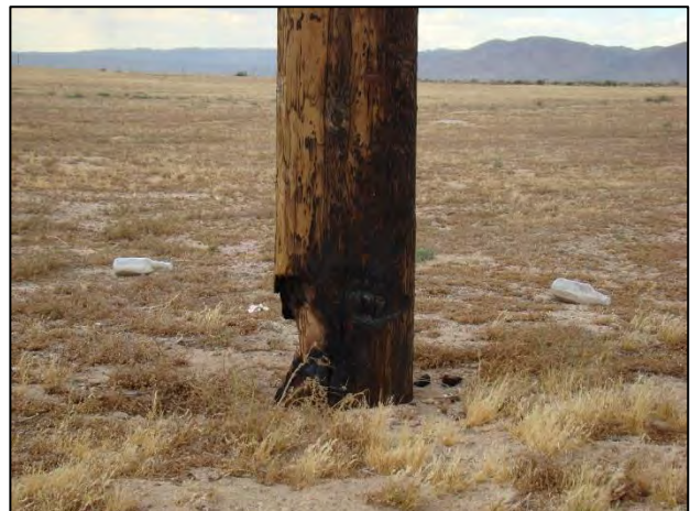
Figure 13-2. Compromised pole discovered during an ARA.
