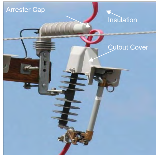
Figure 5-50. Protected cutout/arrester combination.
