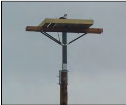
Figure 9-7. Osprey nesting on platform attached to pole-top extension.
