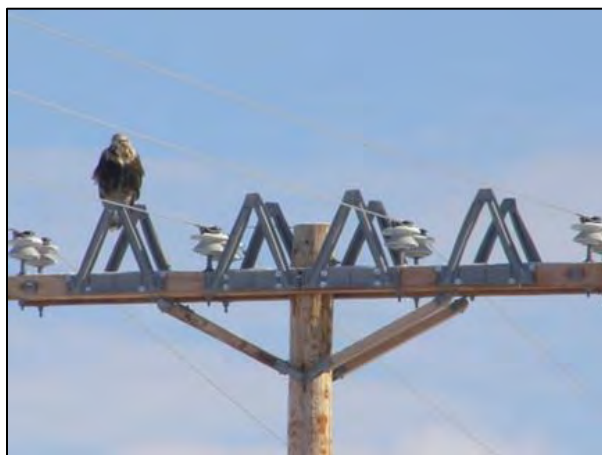
Figure 5-103. Bird perching on a perch discourager.
