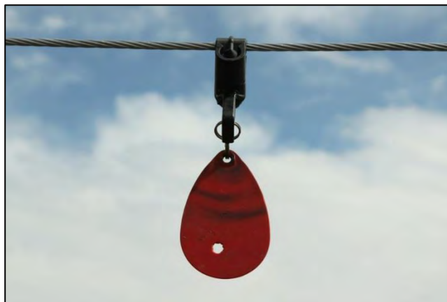
Figure 8-18. Flapper-type marker with a bullet hole.
