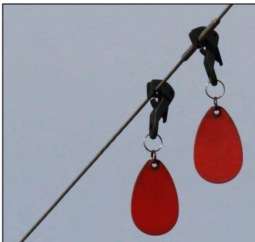
Figure 8-26. Flapper-type markers that have shifted.
