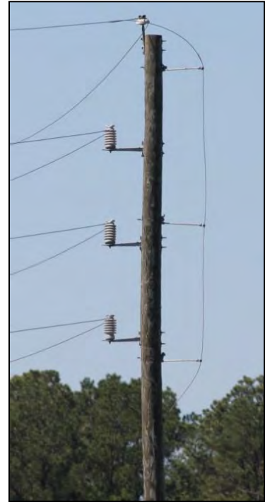
Figure 6-9. Ground wire routed to isolate from conductors.
