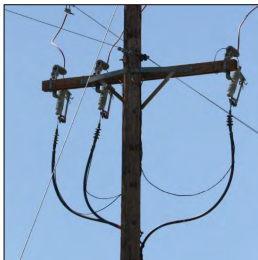
Figure 5-72. Potheads suspended from cutouts.
