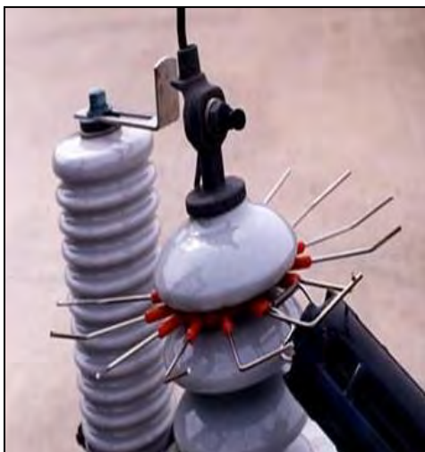
Figure 5-47. 3M Electrostatic Animal Guard.
