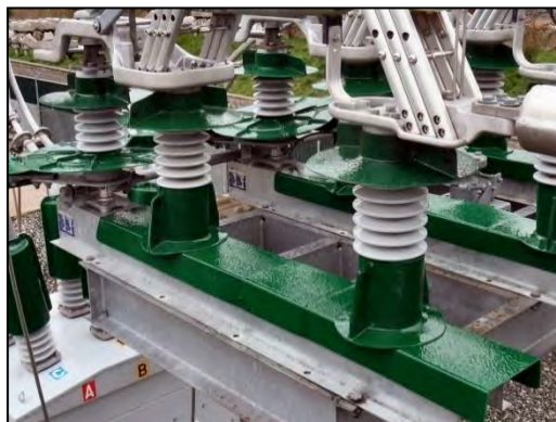
Figure 5-81. Switch with custom-formed barrier plates.
