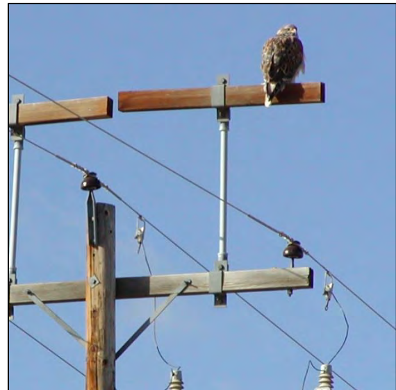
Figure 5-94. Elevated perch encourages birds to use a safe location.
