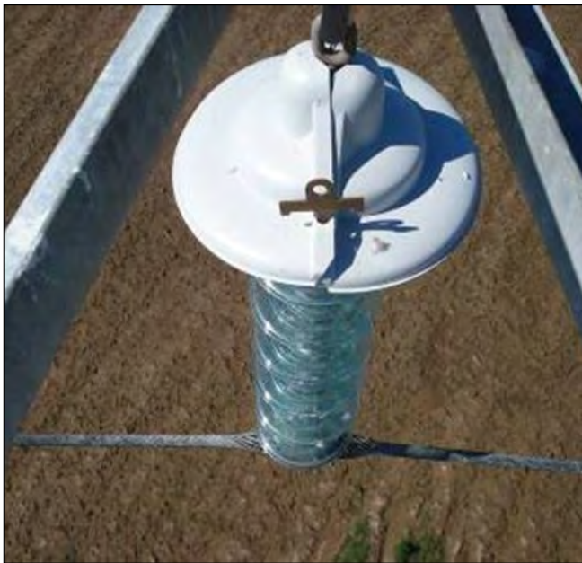
Figure 10-14. Bell insulator stream shield (Kaddas).
