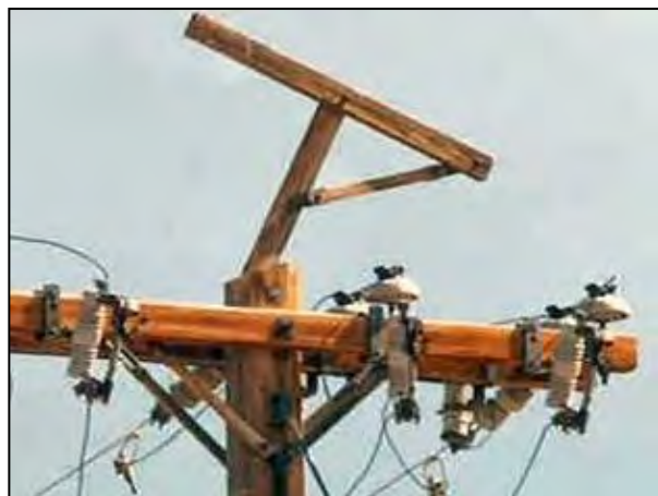
Figure 5-99. Improperly installed elevated perch and unprotected pole.
