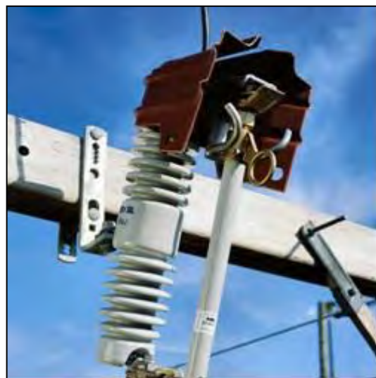
Figure 5-51. Cutout cover (TE Connectivity).
