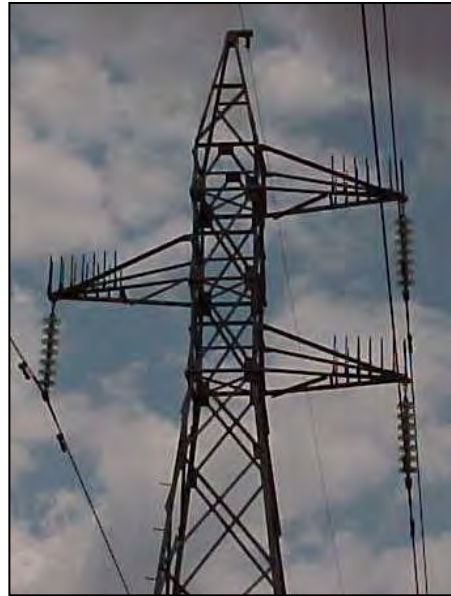
Figure 10-2. HDPE spikes deployed on the arms of a lattice transmission structure (Mission Engineering).
