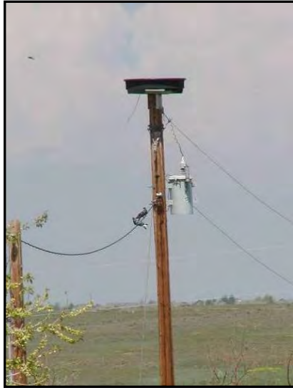
Figure 9-4. Nesting platform above a retrofitted single-phase pole.
