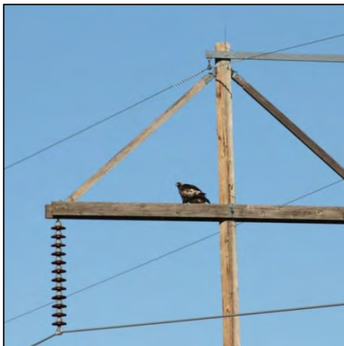
Figure 6-1. Horizontal H-frame tangent structure is safe for perching birds.
