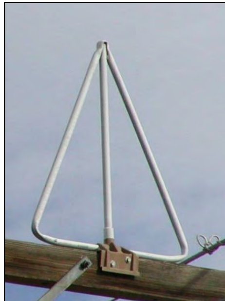
Figure 5-102. Kaddas perch discourager design deters perching within the triangle.
