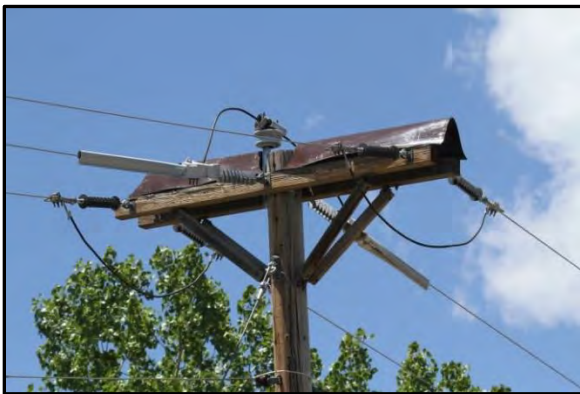
Figure 9-12. Stick deflector prevents nesting materials from being anchored between double crossarms (Power Line Sentry, LLC)
