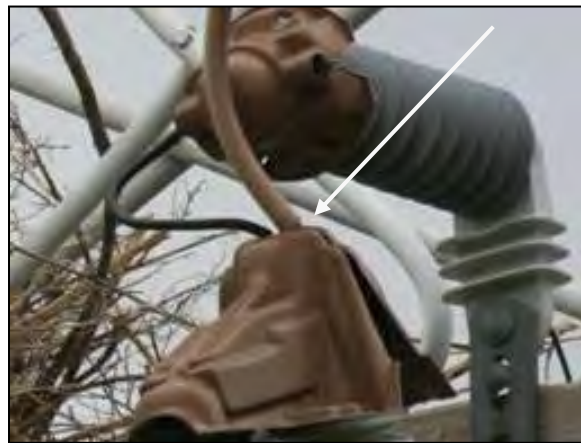
Figure 5-36. Cutout cover with gap between top of cover and bottom of stinger insulation.
