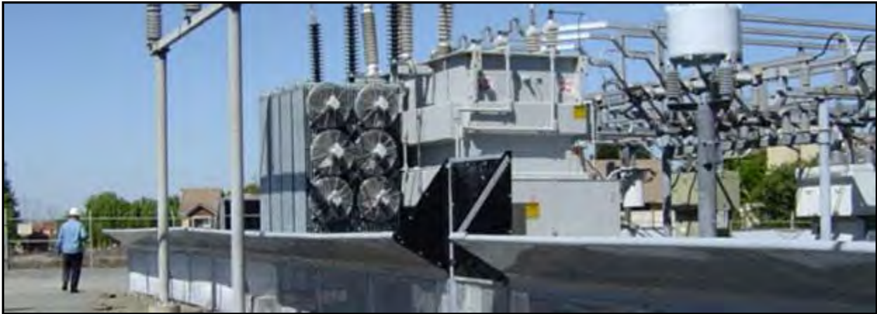
Figure 7-19. Kinectrics PowerKage (Kinectrics).
