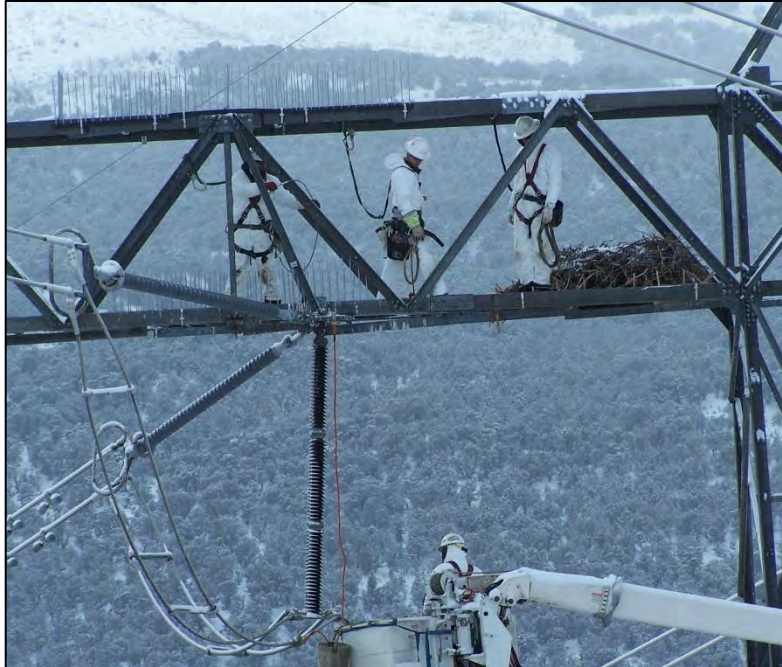
Figure 10-4. Raptor Guard Spike Perching Excluders being installed to prevent perching and defecation on transmission insulators (Power Line Sentry, LLC).
