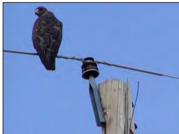
Figure 5-83. Exposed pole-top ground wire
