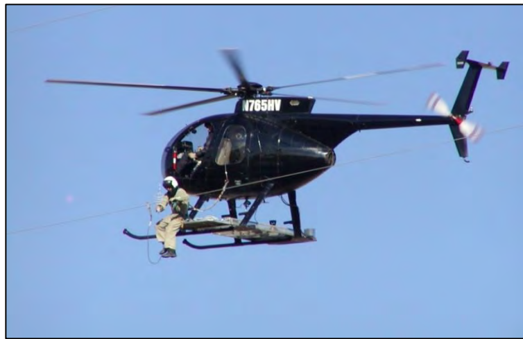
Figure 8-6. Marker installation by helicopter.
