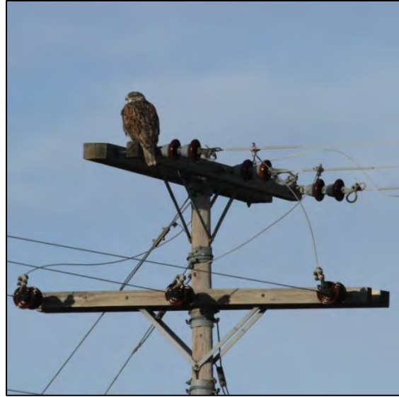
Figure 5-92. Guy wires attached to grounded pole bands.
