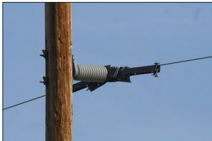
Figure 6-6. Conductor cover for sub-transmission retrofits (TE Connectivity Ltd.).
