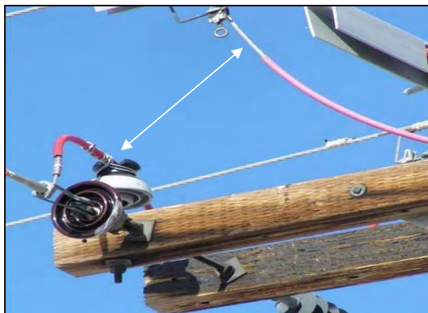
Figure 5-37. Covered jumper with an exposed contact point.
