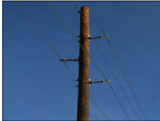
Figure 5-18. Vertical tangent unit (grounded).
