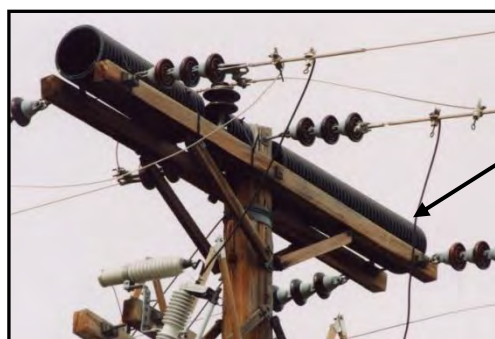
Figure 9-19. Homemade conduit stick deflector.
