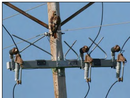
Figure 5-87. Three-phase fiberglass arm with covered cutouts, arresters, and stinger wires. Perch discouragers provide redundant protection.
