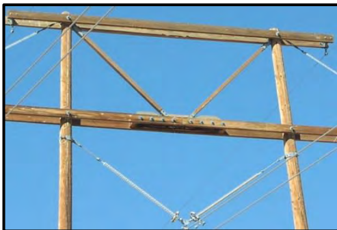
Figure 9-14. Stick deflector (Kaddas Enterprises, Inc.).
