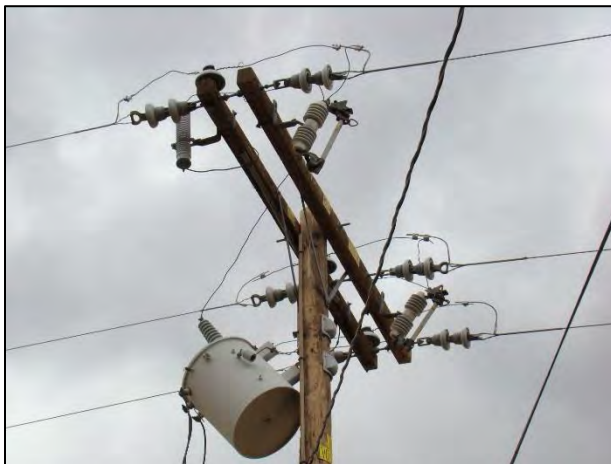
Figure 13-1. Failing transformer mount discovered during an ARA.
