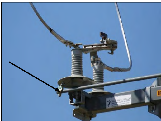
Figure 5-80. Switch with barrier plate.
