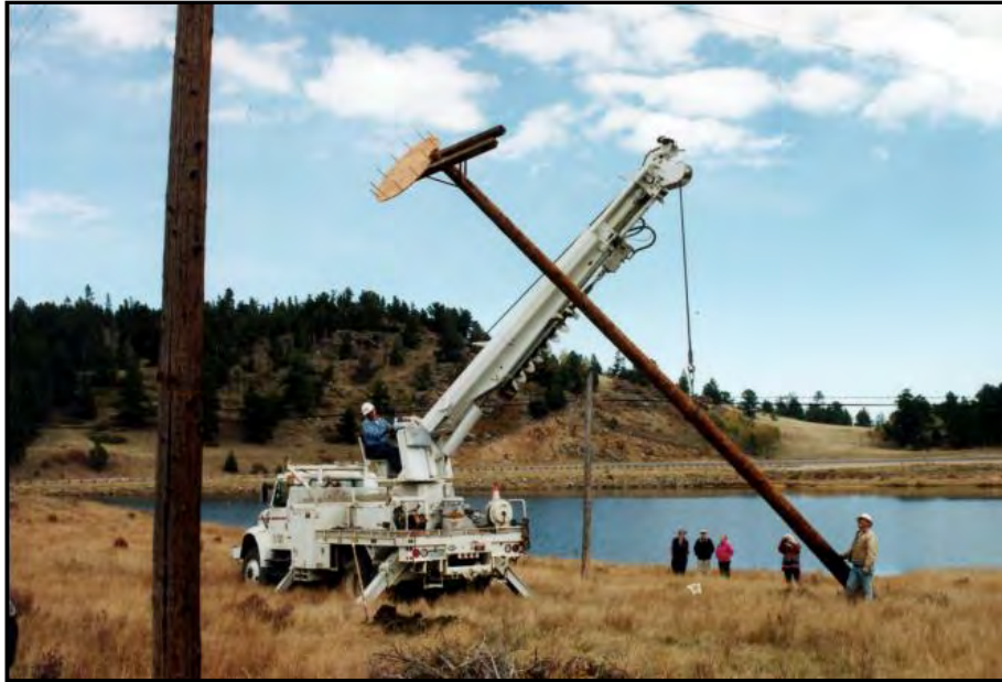
Figure 9-11. Raptor platform with pegs.
