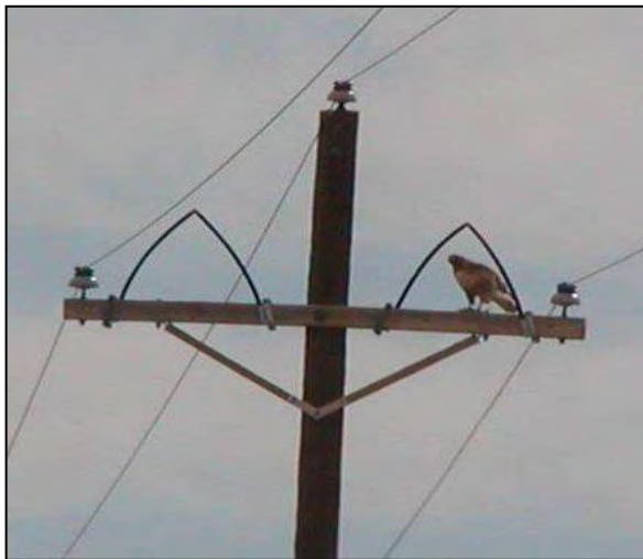
Figure 5-106. Raptor perching beneath a perch discourager.
