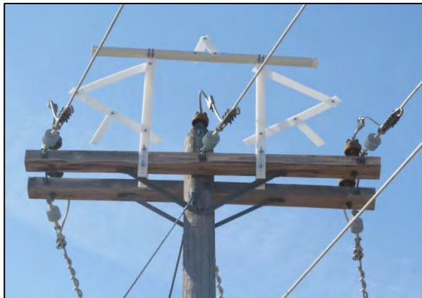
Figure 5-97. Elevated perch (Bird Powerline Protection Ltd.).
