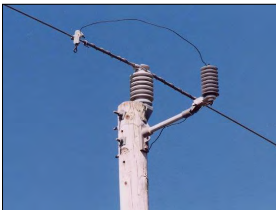
Figure 5-86. Single-phase ungrounded fiberglass bracket.
