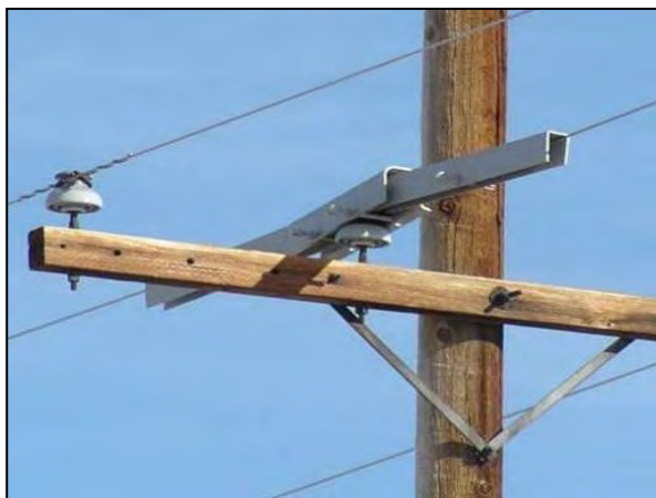
Figure 5-12. Eco Electrical Systems conductor cover.
