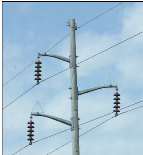
Figure 10-10. Perch discouragers designed to shift large birds away from the insulators.
