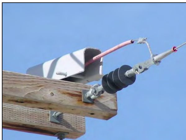
Figure 5-39. Jumper isolated with a pin cover.
