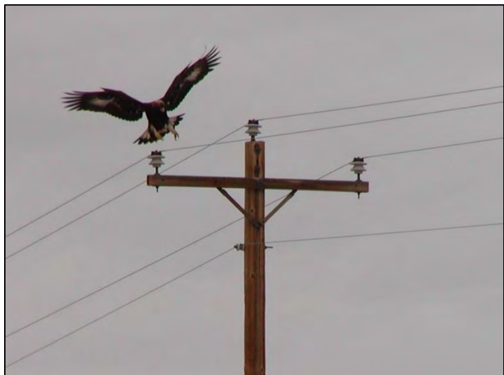
Figure 2-2. Example of Golden Eagle wing span relative to clearances between phase wires on a typical three-phase distribution structure.
