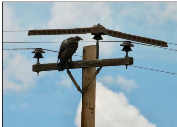
Figure 5-13. Kaddas Enterprises, Inc. conductor cover.
