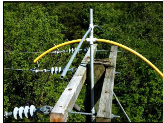
Figure 9-13. Stick deflector restricts the area to build a nest and flexible tubing makes an unsteady perch (Power Supply Company)
