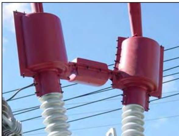
Figure 5-76. Regulator with bypass arrester cover (TE Connectivity).
