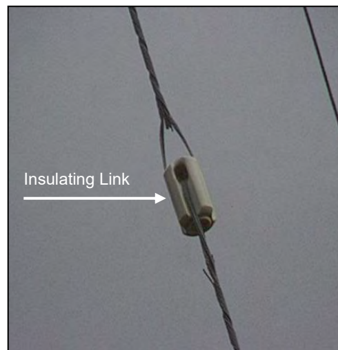
Figure 5-90. Insulating link to prevent a pathway to ground.
