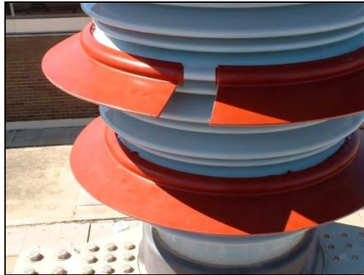
Figure 6-10. Creepage extenders (shown here in a traditional substation application) can also be deployed as barriers on line post insulators.
