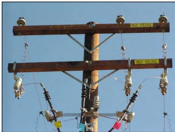
Figure 5-65. Unprotected potheads on a riser pole.
