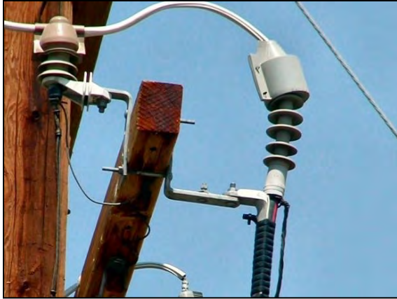
Figure 5-68. Protected riser pole (Salisbury by Honeywell).
