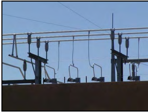
Figure 7-2. Substation bus supports for animal protection.
