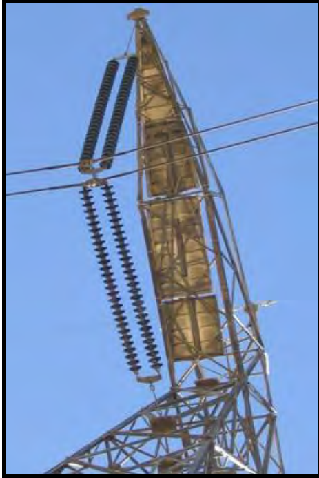
Figure 10-12. Lattice structure with contamination shields (Zena).
