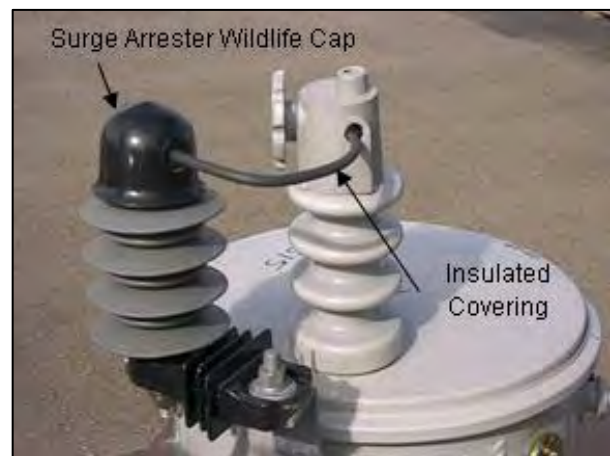
Figure 5-57. Transformer mounted surge arrester with wildlife cap.
