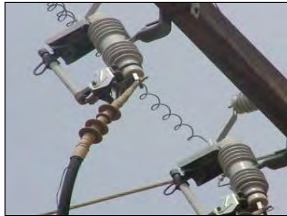
Figure 5-71. Pothead mounted below cutout.
