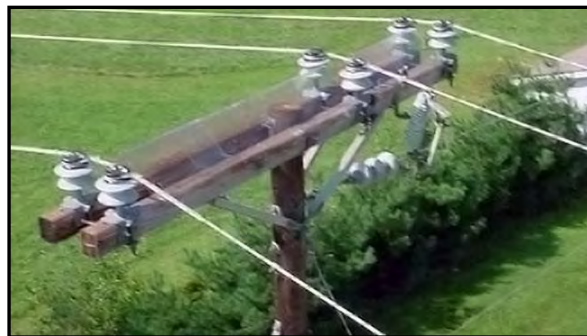
Figure 9-15. Stick deflector (Utility Solutions, Inc.).
