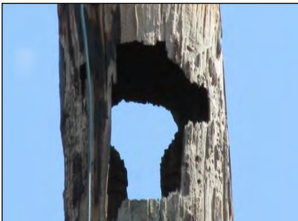
Figure 2-25. Severe damage resulting from Pileated Woodpecker nesting or roosting cavity (Ron Pope).
