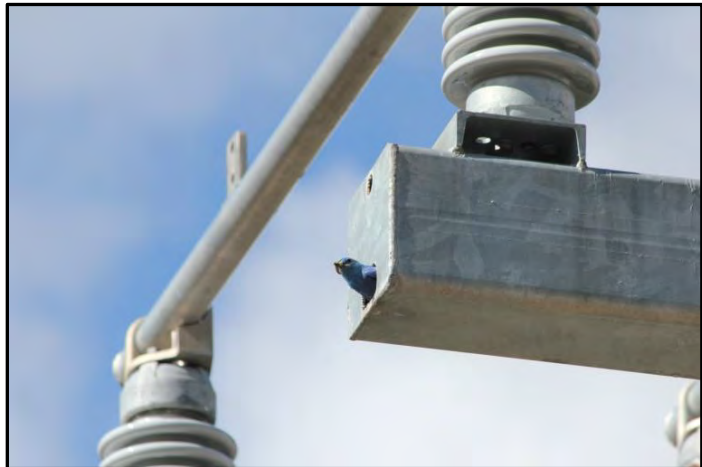
Figure 9-23. Bluebird nest in substation support arm.
