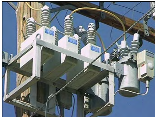
Figure 5-74. Capacitor bank factory-equipped with animal protection.
