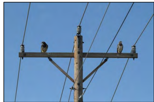
Figure 5-9. Eagle-friendly three-phase pole configuration using a 10-foot crossarm.
