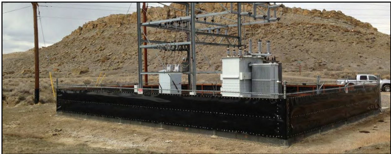
Figure 7-18. Animal-exclusion fence constructed to exclude rodents.
