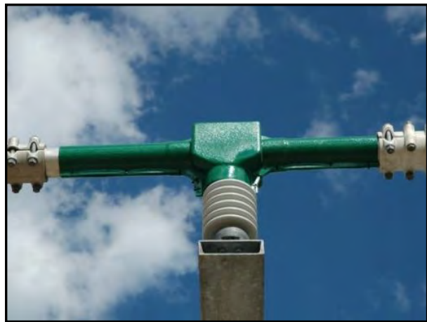
Figure 7-5. Form-fitted bus insulation (Cantega Technologies, Inc.).
