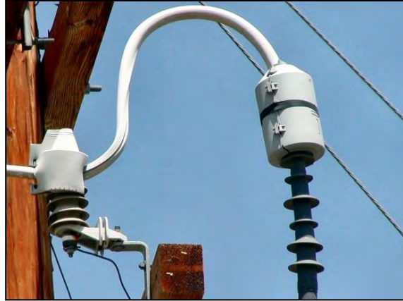
Figure 5-69. Protected riser pole (Hubbell Power Systems, Inc.).
