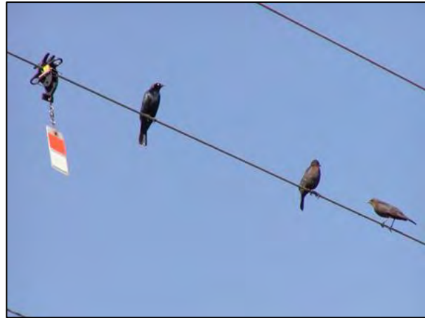
Figure 8-4. Birds perched next to spinning diverter.
