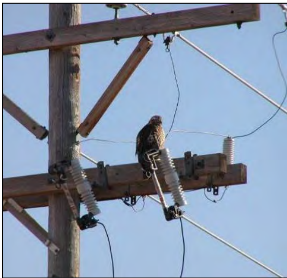
Figure 5-49. Hawk perched between unprotected cutouts and arresters.
