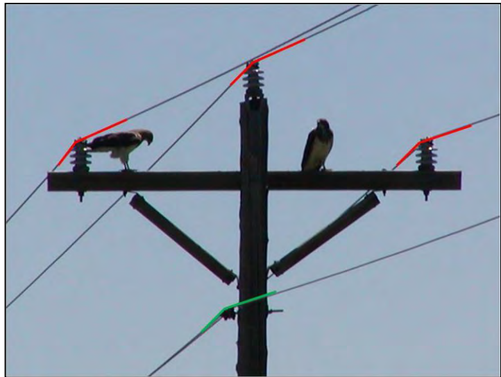
Figure 2-5. Hawk-friendly pole has adequate separation between energized (red) and grounded (green) components.
