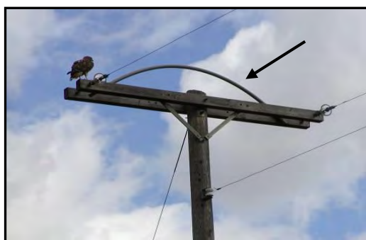
Figure 9-18. Homemade PVC stick deflector.
