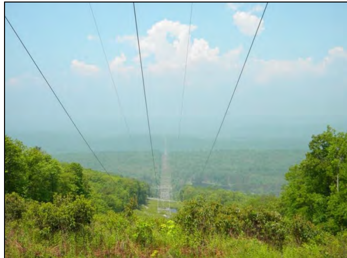
Figure 2-16. OHS wires are less visible than conductors.
