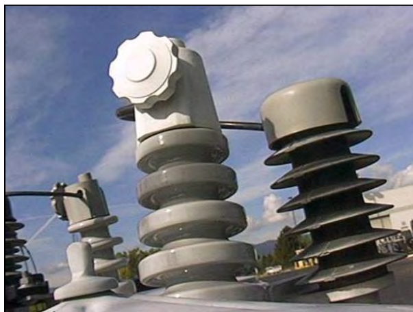
Figure 5-41. "Wheel-type" bushing cover from the manufacturer.
