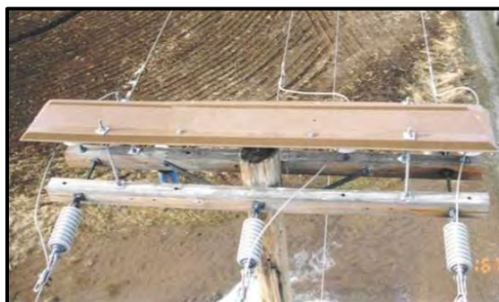
Figure 9-17. Stick deflector specifically designed to prevent nesting above the center phase on an H-frame structure (Kaddas Enterprises, Inc.).
